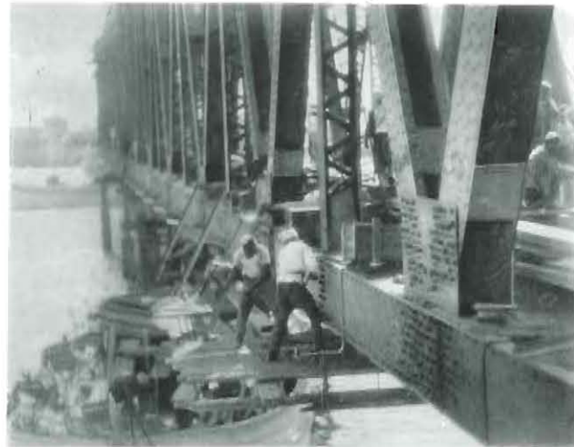
RIVETING SPAN No. 1
