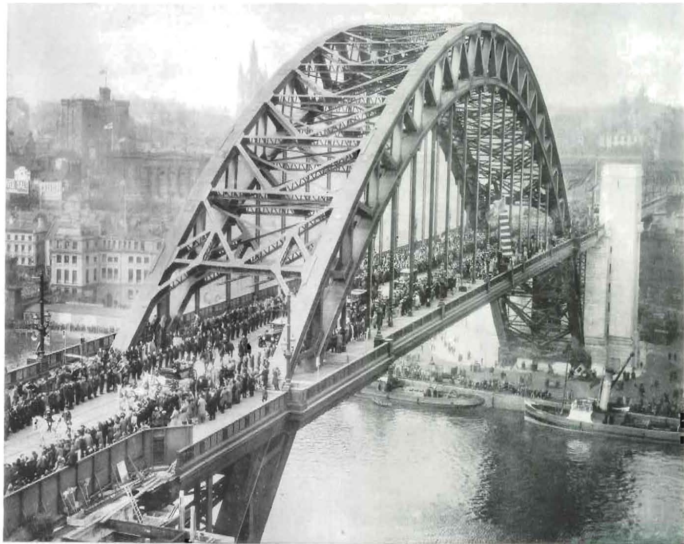
THE OPENING CEREMONY, OCTOBER 10th, 1928. THEIR MAJESTIES THE KING AND QUEEN DRIVING ACROSS THE BRIDGE
