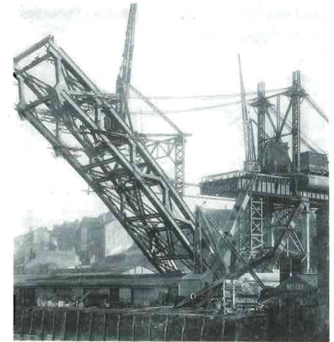
THE ARCH SUPPORTED BY CABLES FROM PANEL POINT 21, WITH THE MASTS AND SECOND POSITION CABLES IN COURSE OF ERECTION.
