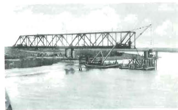
SPAN No 2. UNDER ERECTION, SHOWING TEMPORARY TOP CHORD TIES
