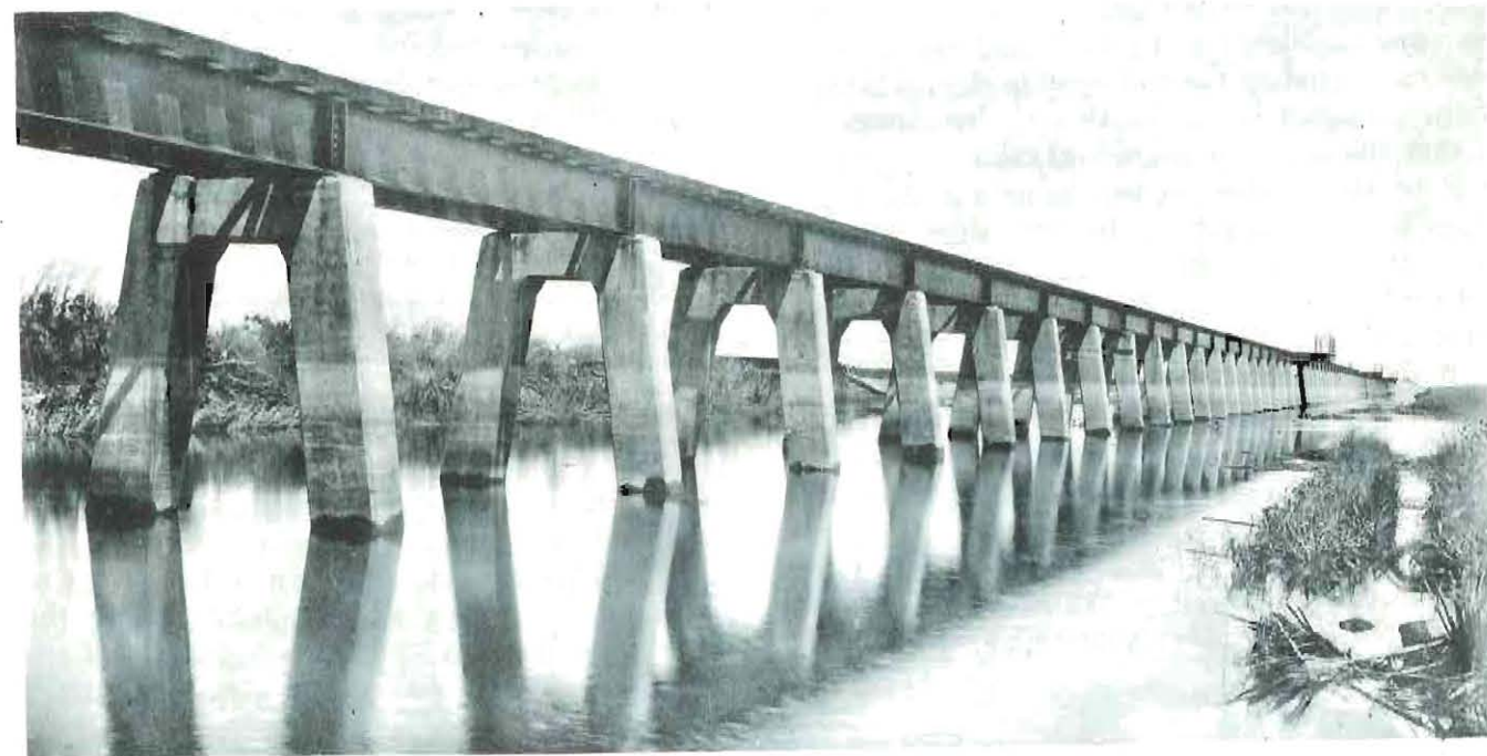
ONE OF THE EIGHT PUNGWE VIADUCTS
