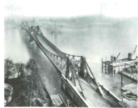
OLD LAMBETH BRIDGE
