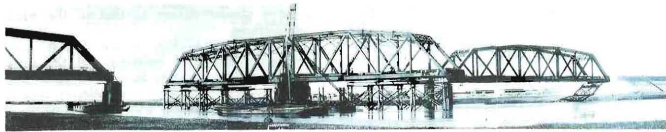
SWING SPAN IN NEARLY-FINISHED CONDITION
