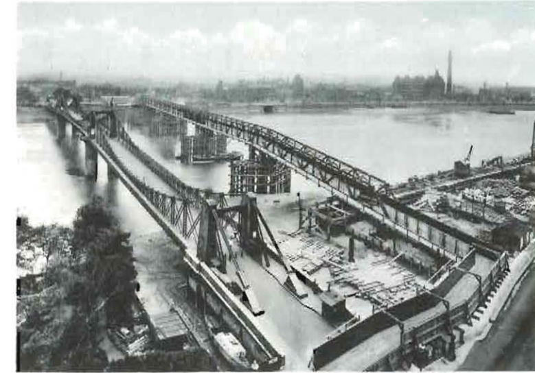
PHOTO TAKEN JUNE 3rd, 1929, SHOWING THE OLD BRIDGE AND TEMPORARY STEEL BRIDGE
